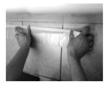
Then, stick masking tape down along the bottom of the tub, so it goes up the tub about 1/8 in.
